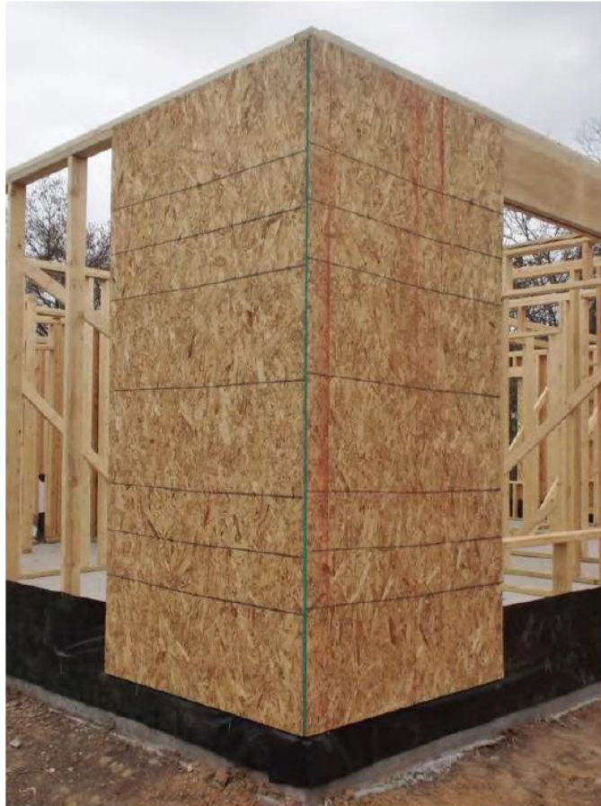
Figure 6-1. Use Full Sheets of Sheathing at Corners
