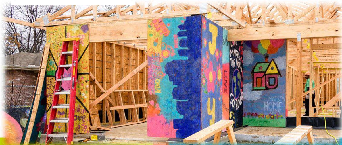
Figure 6-1. Use Full Sheets of Sheathing at Corners
