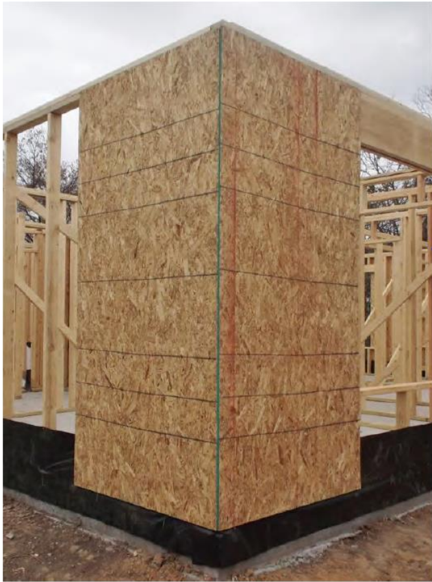
Figure 6-1. Use Full Sheets of Sheathing at Corners
